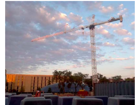
Construction is underway on the Eckhardt Center
