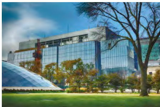
Photo of the William Eckhardt Research Center progressing toward completion
